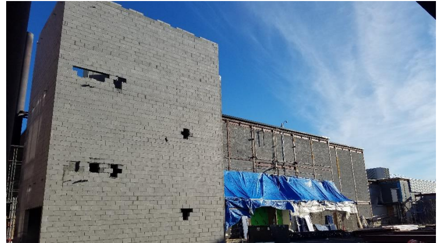
Stair Tower 2-1 (New Addition)
