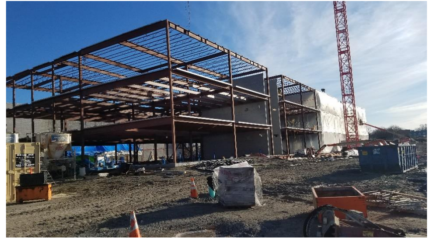
Area 7 & Stair Tower 2-2 (New Addition)
