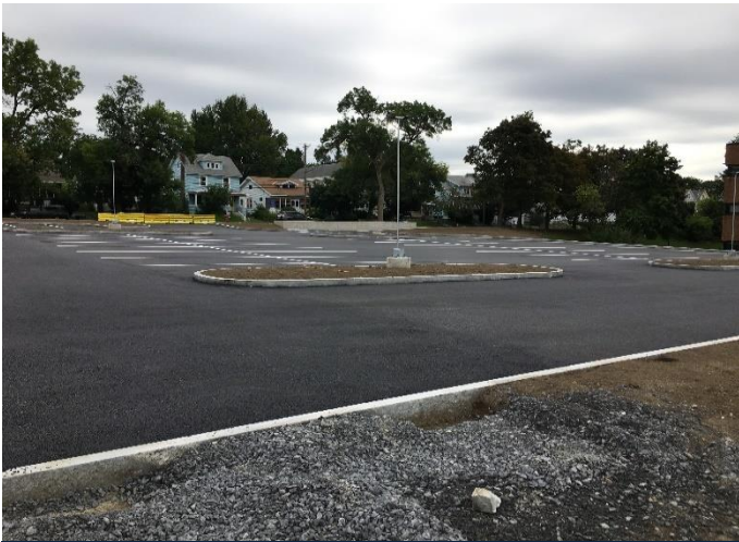
8.31.18—New Parking Lot
