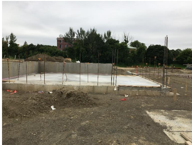
8.31.18— New Stair Foundation
