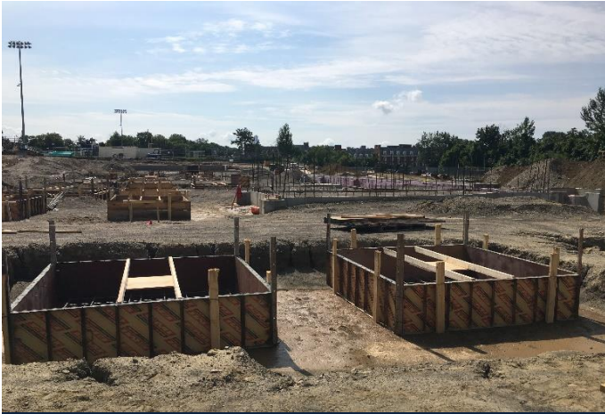
7.31.18—Area 8 (New Addition)
