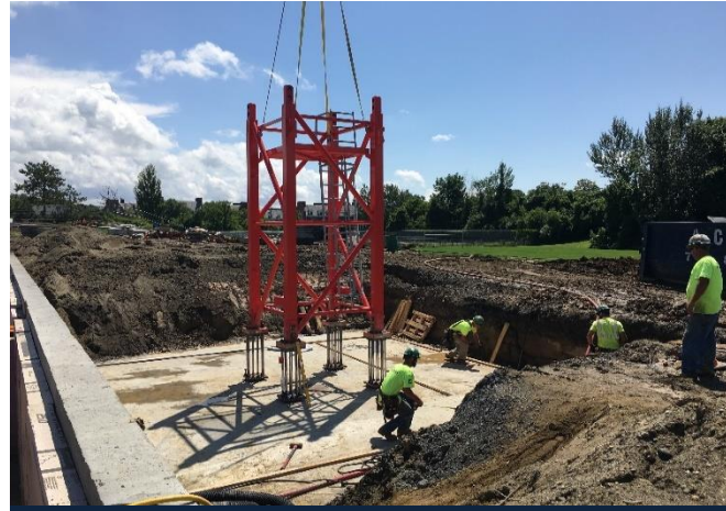
8.14.18—Tower Crane Prep
